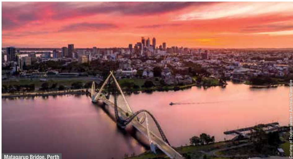
Matagarup Bridge, Perth
